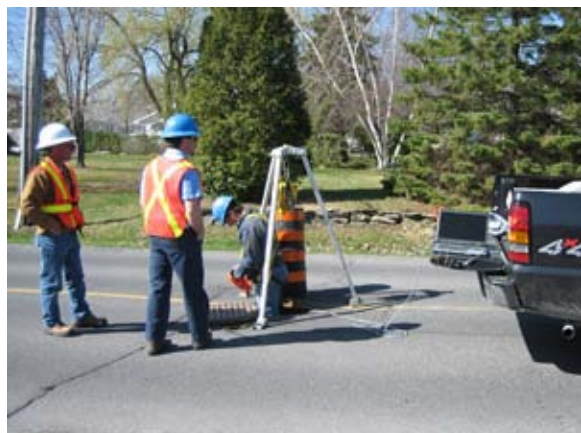
Manhole Location Selected for Flow Survey
