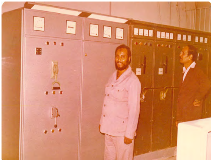
Electrical Boards Installation and Integration Undertaken By Kimans Inc.
