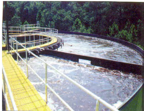
One of the new & improved phases at a water treatment plant.
