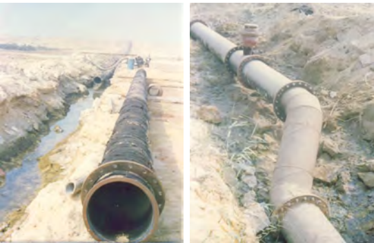
Different Stages Of Pipe Line Networks Supplied & Installed By Kimans Inc.
